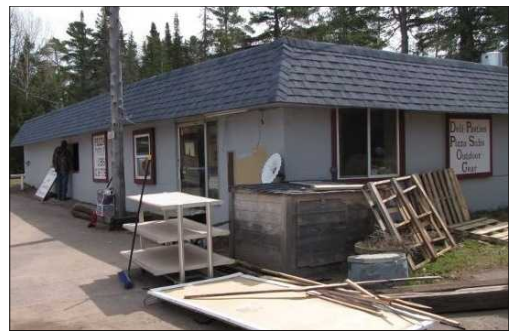
Outside of the old deli, just as work started.
